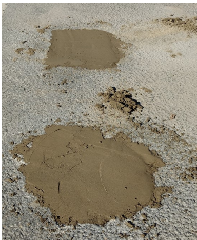
Figure 6: X-Phalt™ very rapid repair mortar placed in both adjacent repairs with 10-15 minutes working time. Opened to traffic in less than 90 minutes.
