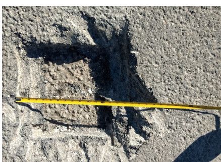
Figure 4: Damaged wear layer area removed down to sound base layer
