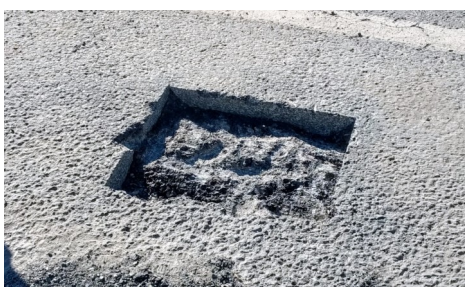
Figure 2: Saw Cut and Prepped Pothole prior to Repair with X-Phalt™
