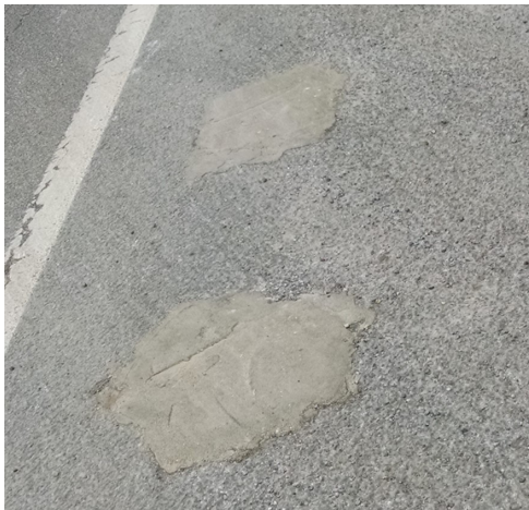
Figure 6: X-Phalt™ very rapid repair mortar placed in both adjacent repairs with 10-15 minutes working time. Opened to traffic in less than 90 minutes.
