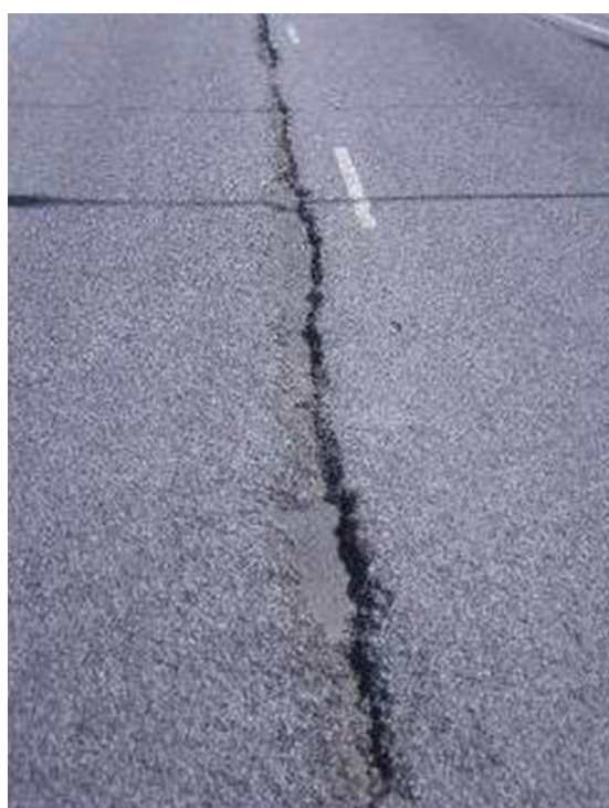
Figure 1: Longitudinal Construction Joint Crack between Lanes. Note the Large Gap Near the Foreground.
