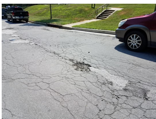
Figure 1: Deteriorating roadway. Note the cracking, distortion and disintegration of the surface and deeper levels.
