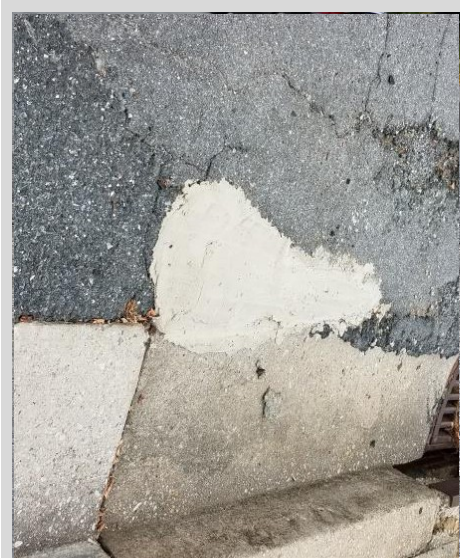
Figure 3: X-PHALT™ pothole repair tenaciously bonding to both asphalt and concrete
