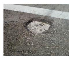
Preparation: remove any loose debris and standing water, dampen the concrete base layer to prevent drawing excess water from the wet X-PHALT<sup>TM</sup> during cure.
