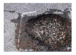
Preferred preparation: saw cut back (or chisel) until sound adjacent top layer and base layer are exposed; remove loose debris and standing water; fill and finish with hand tools to desired texture (trowel, tine or broom finish).
