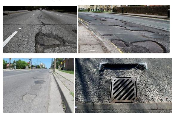
Preparation: if necessary, saw cut back (or chisel) until sound adjacent top layer is exposed; remove loose debris and standing water; fill and finish with hand tools to desired texture. Note: if there are any existing cracks in the base layer, they may reflect through the cementitious repair. However, the chemical bond between X-PHALT<sup>TM</sup> and the asphalt will keep the repair in place and attached to the asphalt base course.
