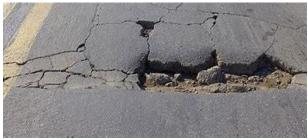
Preparation: remove loose debris; remove damaged material around the perimeter, <u>chisel away</u> all sharp points jutting from the bottom and side to remove stress concentrators that will initiate <u>cracks</u>; fill with repair material and finish with desired texture. Note: the sub base must be firm enough to support the loading transfer from the repair material without deflection.
